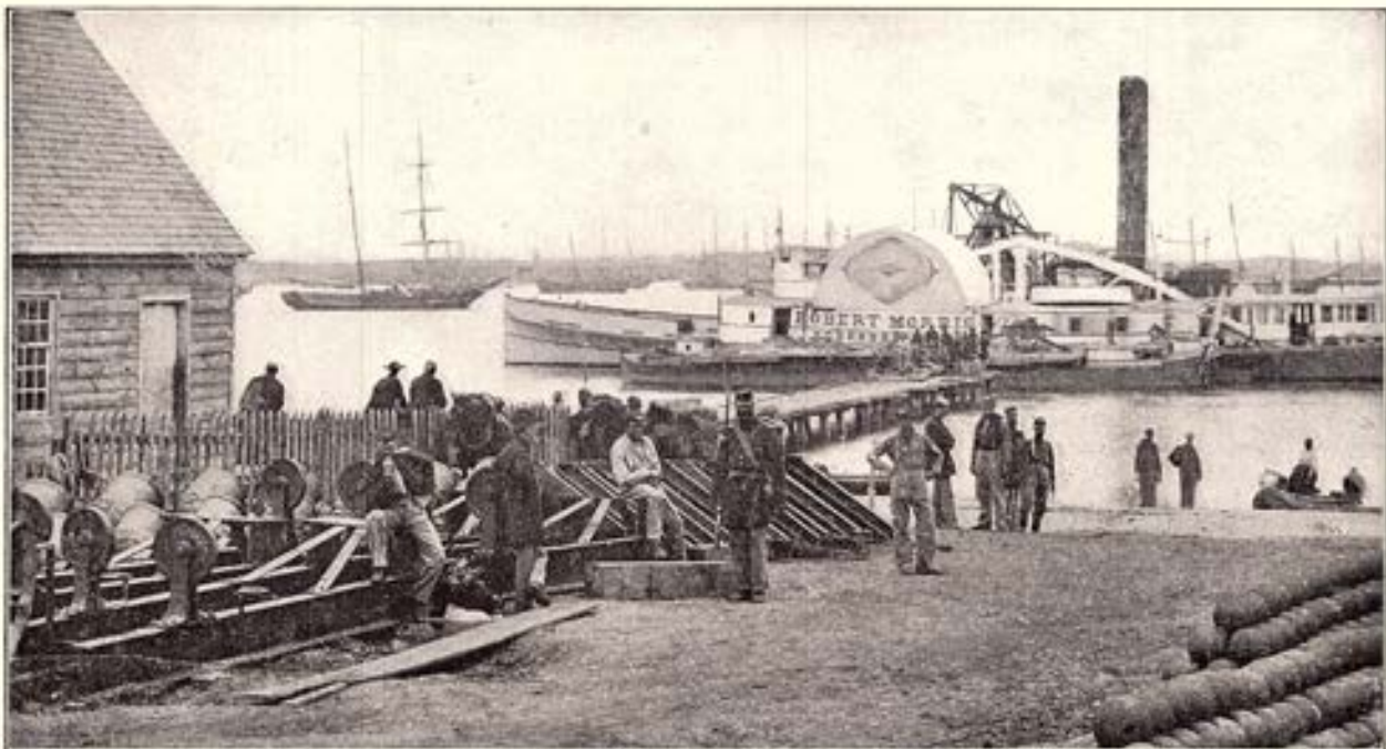
LOADING THE TRANSPORTS
