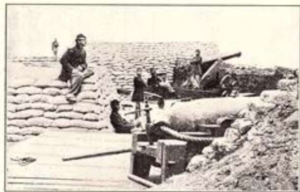
GUNS THE UNION LOST AND RECOVERED. (A two-gun Confederate battery in the entrenchments south of Yorktown.) The near gun is a 32-pounder Navy gun which had been burst, wrecking its embaseure. The far one, a 24-pounder siege-piece. More than 3,000 pieces of naval ordnance fell into the hands of the Confederates early in the war, through the ill-advised and hasty abandonment of Norfolk Navy Yard by the Federals. Many of these guns did service at Yorktown and subsequently on the James River against the Union.
