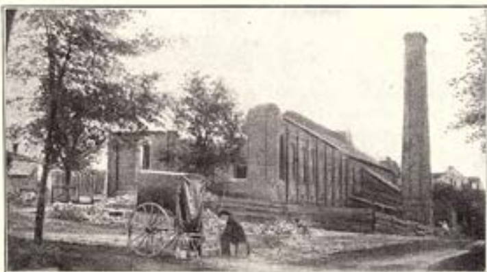
RUINS OF STATE ARMORY, COLUMBIA, 1865
