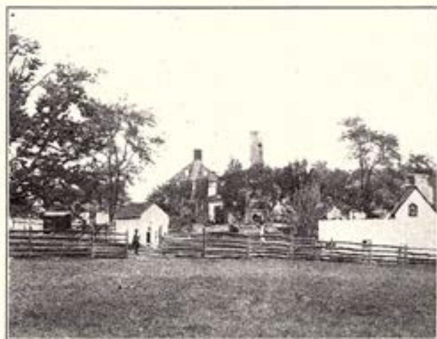
RUIN OF MUMMA'S HOUSE, ANTIETAM
