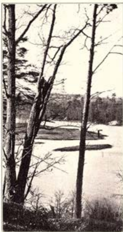
BUTLER'S SIGNAL TOWER
