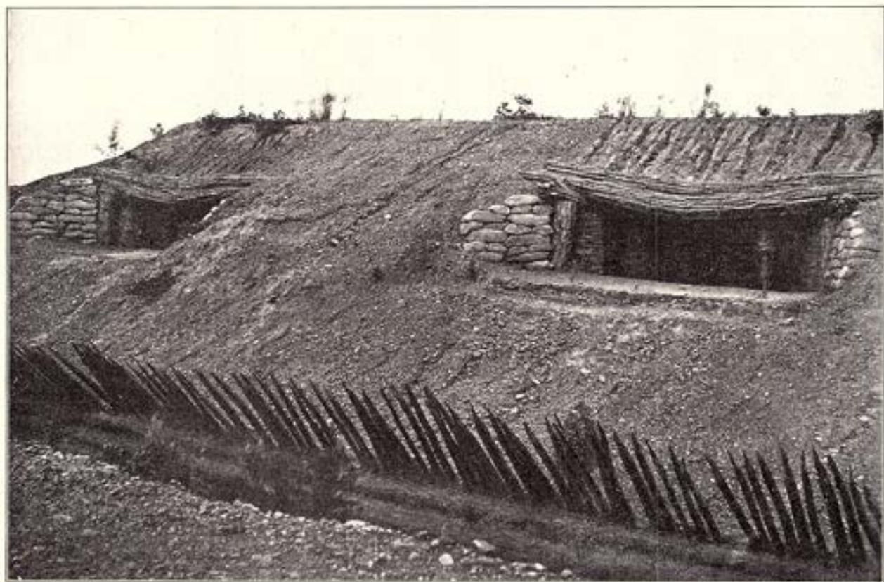
PALISADES AND PARAPET AT FORT HARRISON
